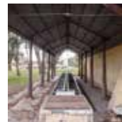
Nuraminis, Lavatoio Is Muracelus, 1932-33 (foto F.S.)
