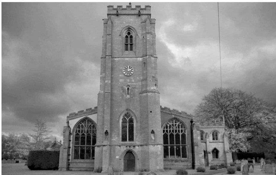
Fig. 3.9: The west front of the parish church of Walpole St Peter, Norfolk. Clear distinctions between architectural phases are visible with the original tower, constructed in c.1300, the later nave dating to the 1360s and the later south porch (c.1425) on the right-hand side. Photograph by the author.
