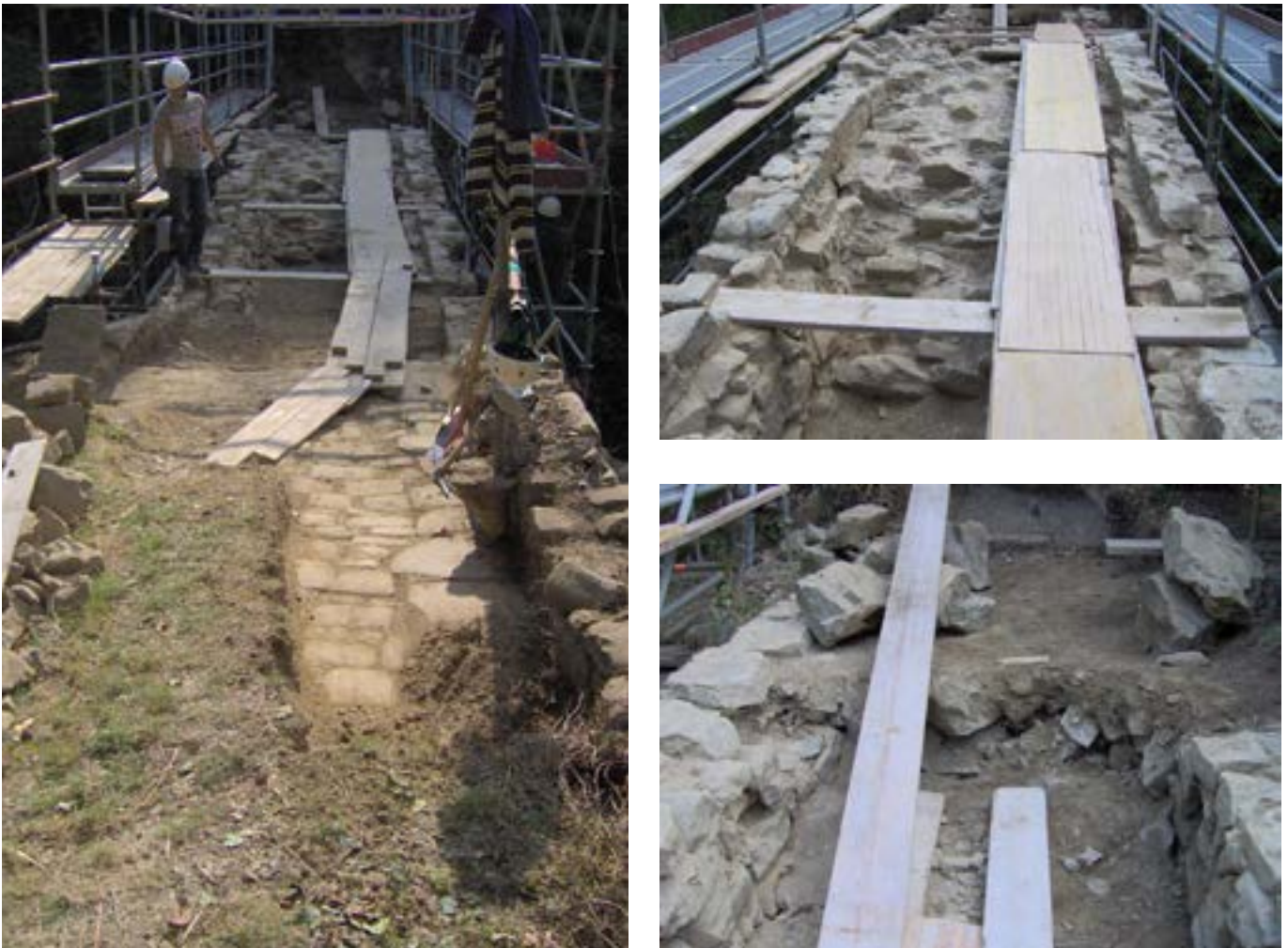
fig. 2, Ponte in restauro
